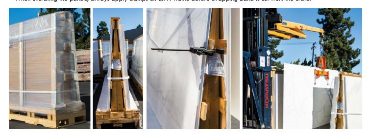
• Use a forklift boom & pitch clamp to carefully move the panels from the original slim factory A-frame, to an A-frame with a wider base and more obtuse angle. We recommend padding the A-frame prior to placing the panels on to each of its sides.
