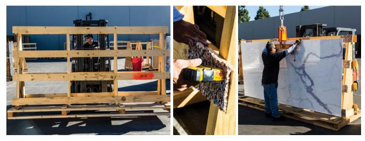
• Use 3 straps to tie the panels to the A-frame, and wrap plastic around the entire A-frame 3X to prepare the package for shipment.
